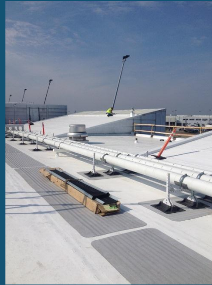
Concourse D Roof Replacement
